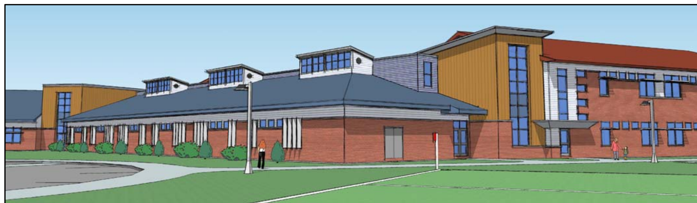
3 KINDERGARTEN WINGS LOOKING TOWARDS STAIR LOBBY
